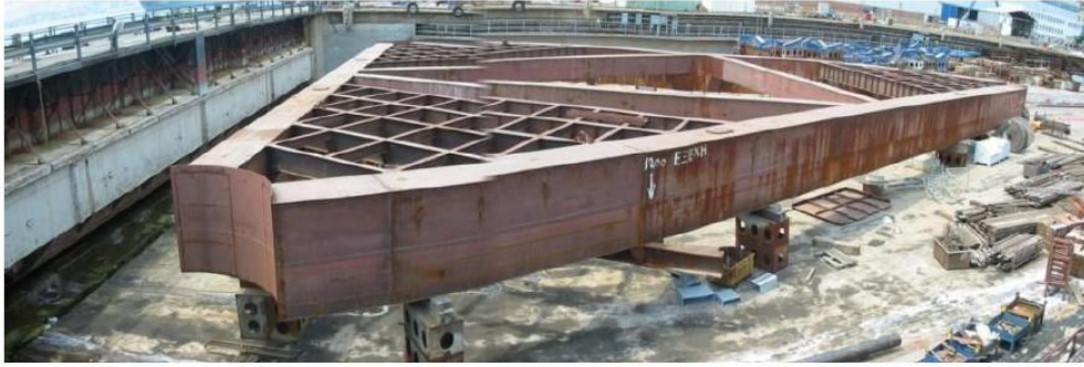
Fig 1.6. The triangle structure and reinforcements after construction (mosaic of a couple of photographs due to the large size).
