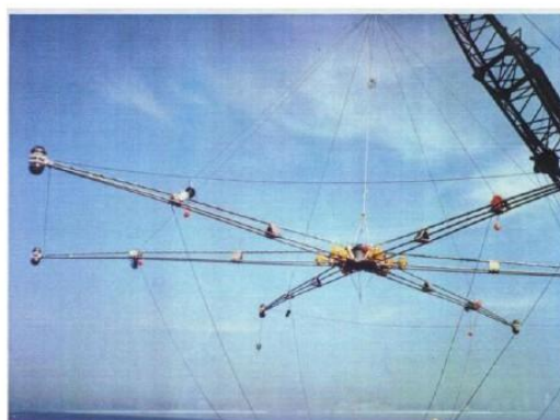
Fig. 1.1b. The aluminium floor, constructed out of aluminium alloy pipes
