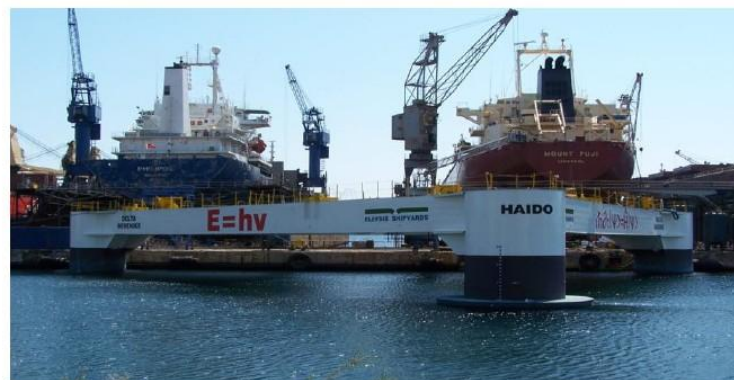
Fig 1.11b. Painted and ready to install the ancillary equipment
