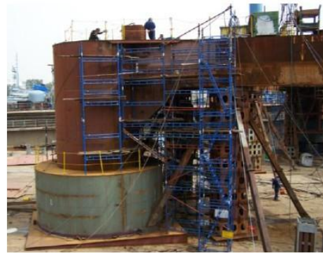
Fig 1.8. Welding a cylinder to the triangle
